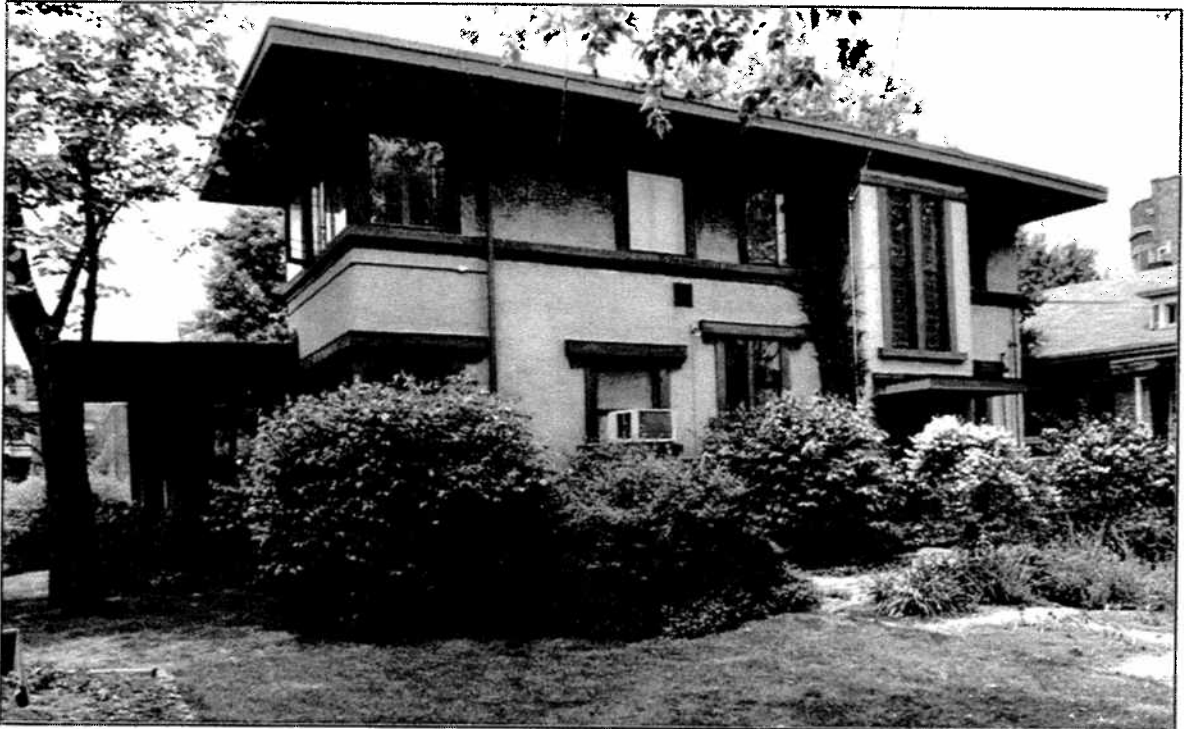
The rear (east) elevation of the Miller House demonstrates the manner in which Prairie architects "broke the box" of traditional architectural forms. The placement of windows at the corners of the house is in contrast to the conventional expectations of corners as solids. Note also how the direct expression of the stair hall breaks the flat wall plane. ( Raymond T. Tatum, photographer )
